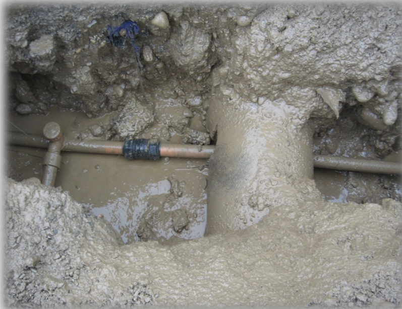
Unlocatable storm sewer with an intersecting gas line -- This is a classic Example of a “Cross-Bore”.
