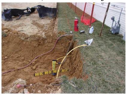
Another example of overlooking "clear evidence" prior to excavation! The gas meter was clear evidence that an underground facility was in direct proximity to the dig.
