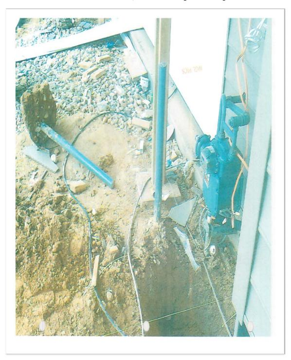
During this deck installation, the Contractor removed the bollard protecting the gas meter in order to auger a hole for a deck support, violating §12-127(e), the "Clear Evidence" section of the statute.
