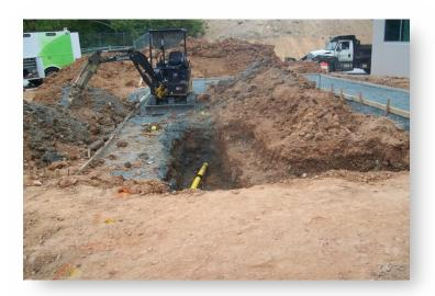
This contractor not only violated the mechanical equipment section of the law §12-127(c), he also drilled a hole in this gas main (yellow pipe) to see if it was pressurized.
