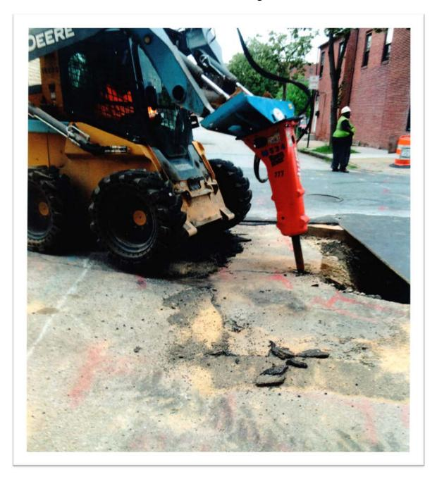
Violation of  $\S12-127(c)(2)$  - Using Mechanical Equipment within 18" of the Tolerance Zone and within 18" of the Marks. Below this 6000psi hammer was a 115,000-volt electric cable.
