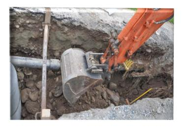
Yes! Using mechanized equipment within 18" of an underground facility is a violation of  $\S12-127(c)(3)$ .
