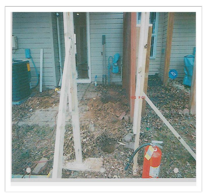
Deck installations cause a multitude of damages to underground facilities in Maryland! This is a violation of §12-124 (Failure to call Miss Utility) and §12-127 (Clear Evidence.) This deck installer did not have a "Miss Utility" ticket and was digging immediately in front of a gas meter...!
