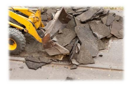
Yes! Removing Asphalt or Concrete without a Miss Utility Ticket is considered excavation activity and is a violation of Title XII which is a violation of §12-127(c) - Using mechanical equipment within 18" of an underground facility.
