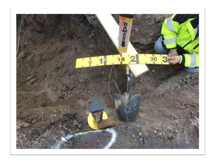
This is an example of a "hit kit" which is used to identify the damaged area during a typical investigation. The damaged gas service line lays under the tolerance zone measure, the white paint circle shows where the original red mark for electric service was at the time of excavation. The violation in this photograph is digging within the 18" tolerance zone \$12-127(c)(2).
