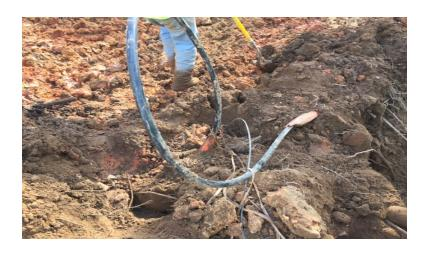
This an example of what can happen when a facility is mis-marked. The high-profile communications line in the photo was marked 12 feet in error, causing the contractor to damage the line. Very costly to repair and very disruptive to customers.
