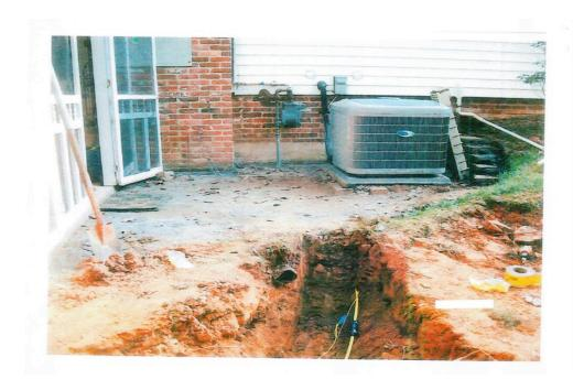
The damage to the gas service line in this photo could have been avoided if the contractor has paid attention to the "clear evidence" (§12-127) on this job site. The gas meter was an excellent clue to where the gas service was entering this building. Had they called Miss Utility, the gas line would have been marked. Without location marks, the contractor should have called in a discrepancy, since the gas meter clearly showed a buried service existed.
