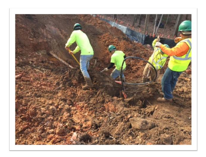
This major communication conduit was severely damaged due to the violation of §12-126, "failure to properly locate an underground facility." The violator was billed \$150,000 by the facility owner and was fined by the Authority as well."- Non-compliance of the Title XII statute can be very costly.
