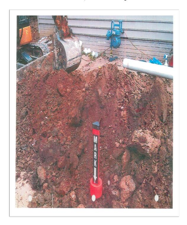
This is the 3<sup>rd</sup> violation for this Contractor. He did not have a "Miss Utility" Ticket and was operating mechanical equipment within 18" of a utility and ignored the "clear evidence" - a gas meter attached to the side of the residence.
