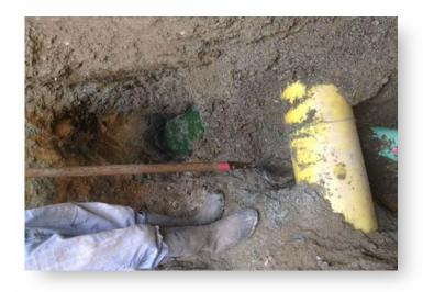
This is a photograph of a gas main (yellow pipe) cross-bore through a WSSC sewer main which was discovered in late 2017. Situations like these can cause catastrophic events, if not detected in a timely manner.
