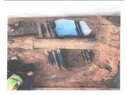
Five (5) large gas service lines were cross-bored through an unlocatable residential water main... the danger from these occurrences have a very real potential for catastrophe!
